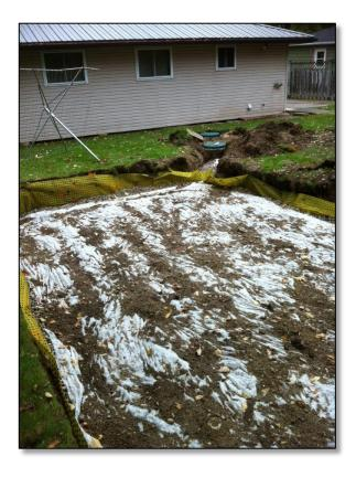
With each roll of BIOBARRIER, plastic pegs are provided that are used to secure the BIOBARRIER near the surface of the soil.
